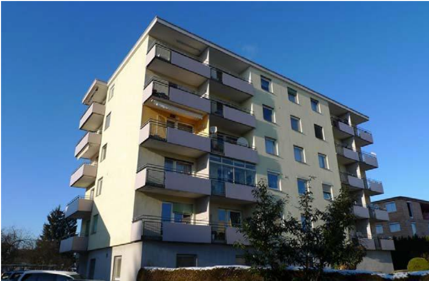
Photo: Dwelling house Bahnhofstr. 43, 6890 Lustenau with ETICS made of EPS (year of construction 1966)
