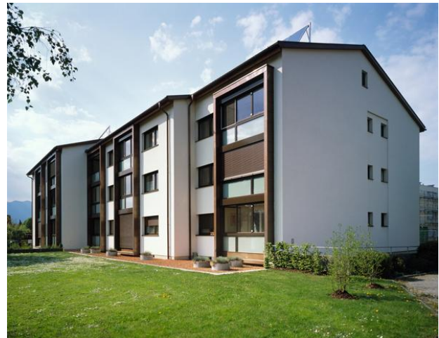
Photo: Dwelling house Rankweil-Schleipweg after renovation
