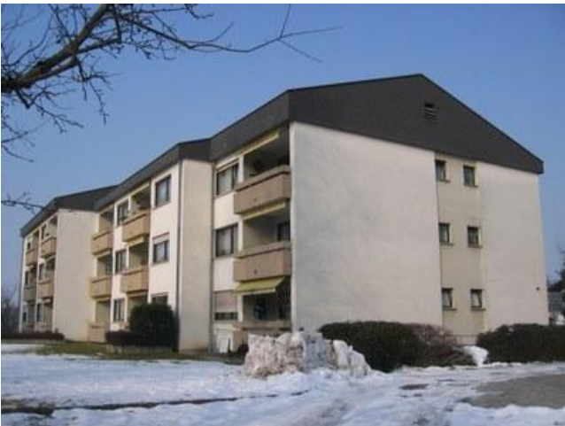
Photo: Dwelling house Rankweil-Schleipweg before renovation
